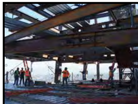
Structural Steel Erection
